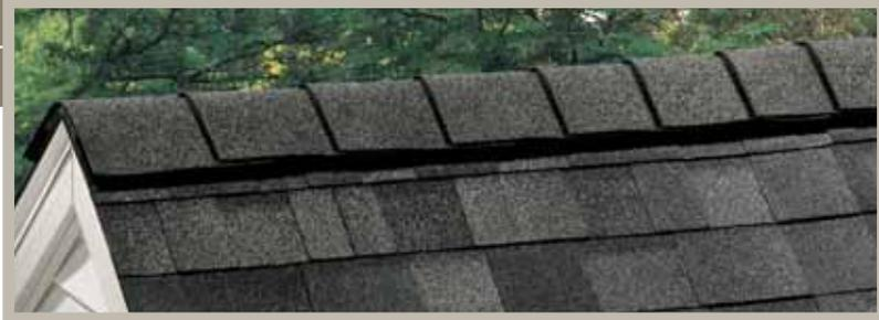
Shingles have two important jobs to do – provide durable protection and complement the aesthetics of your home. **Hip** and **ridge** shingles do those same jobs at the top of each slope while also protecting the ridge vents that allow moist air to escape from the attic.
