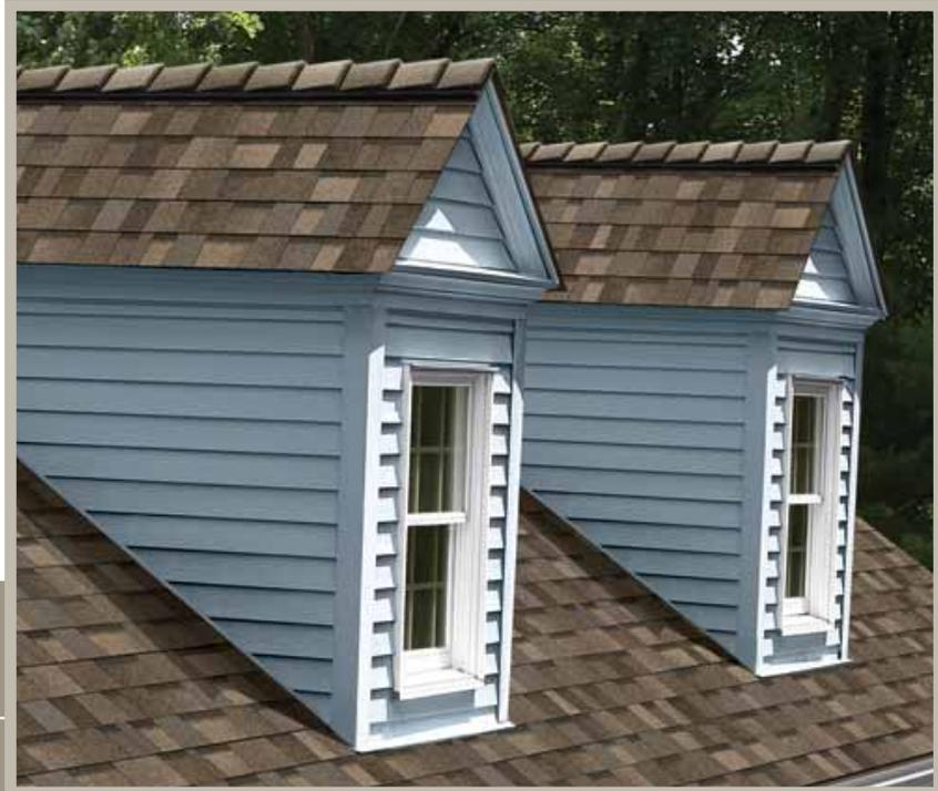
According to an article on DoItYourself.com, not keeping hip and ridge shingles in a straight line is one of the most common mistakes in applying roofing shingles. Pre-cut or pre-scored hip and ridge shingles allow for more uniformity along your roof lines.
